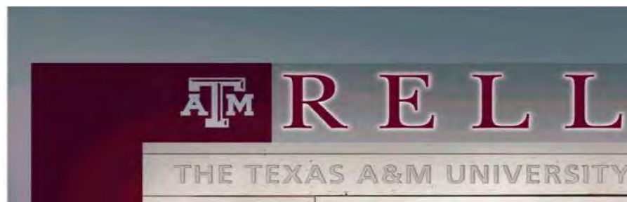
FIGURE 7.12 Primary logo cut out of field with halo illumination. Sub-text relief cut out of stone sign face and lit with external ground lighting. Secondary branding element, cut out of field with white halo lighting.
