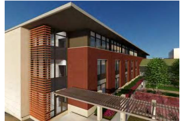
FIGURE 6.38 Horizontal louvers and roof overhangs at the CIR protect large areas of glazing to mitigate solar heat gain.
