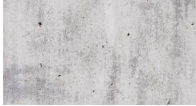
Smooth finished concrete (sign foundation only)
