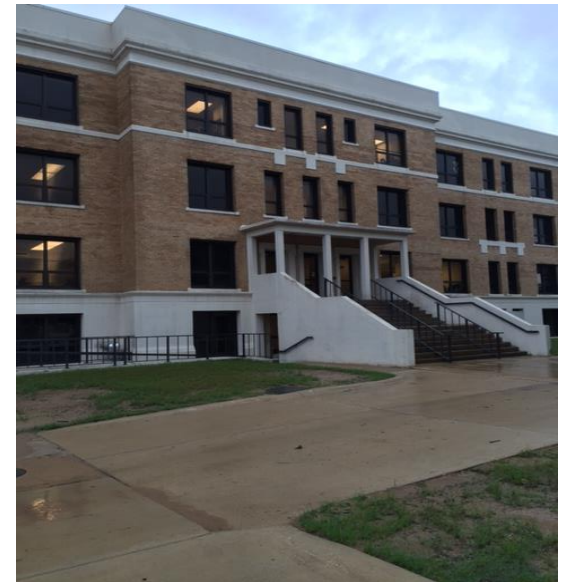
Milner Hall – North Entrance from Northside Parking Garage
